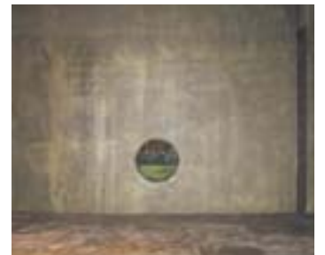
RC薬品貯蔵槽
